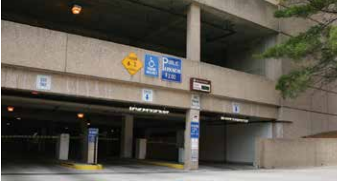
The City Hall parking garage is located under and adjacent to City Hall at 200 N. Second Street. There are entrances to the structure from Monroe and Second Streets.
