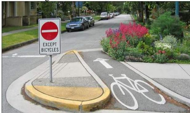
**Closures** - generally on residential streets, these prohibit through-traffic movement or prevent undesirable turns. Street closures may be appropriate where large volumes of through-traffic or “short-cut” maneuvers create unsafe conditions in a residential environment.
